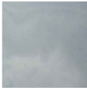
Weathered Concrete Ref: 92
