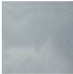
Weathered Concrete Ref: 92
